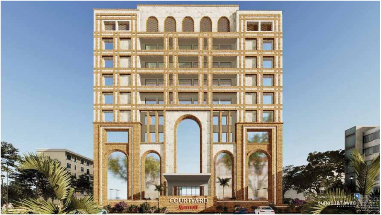
Courtyard by Marriott, Islamabad, S & F Under Construction
