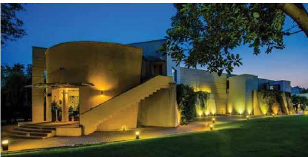
50 meters Swimming Pool and Service Building - Islamabad Club, S & F
