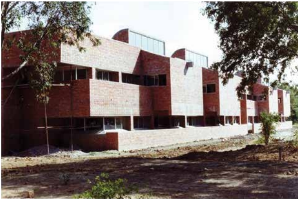
Flying Wing Building, P.A.F Academy, Risalpur 1984-1990, S & P
