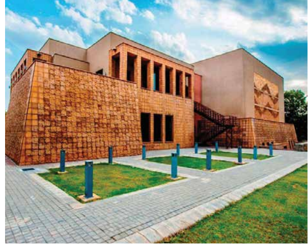
Badminton, Fitness Gymnasium & Table Tennis Building, Islamabad Club, S & P
