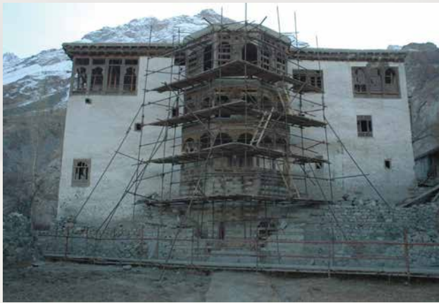
Fig 3: Above Pre conservation façade
