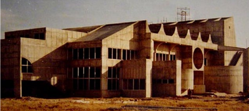
Convocation Hall/Auditorium P.A.F Academy, Risalpur 1984-1990, S & P
