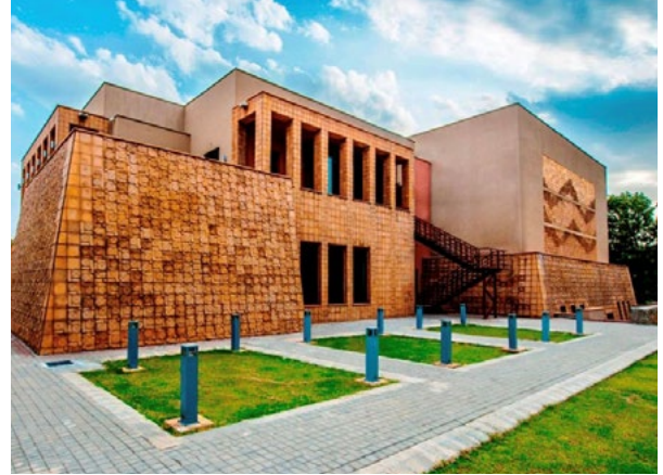
Badminton, Fitness Gymnasium & Table Tennis Building, Islamabad Club, S & P
