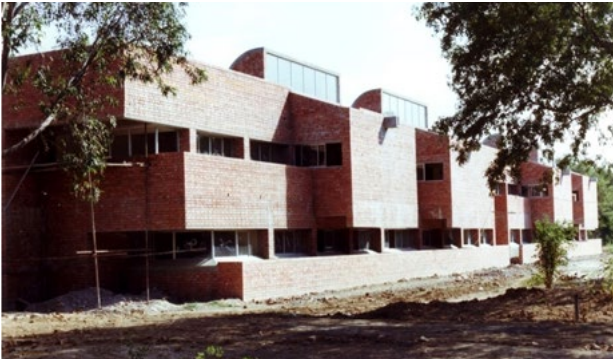
Flying Wing Building, P.A.F Academy, Risalpur 1984-1990, S & P
