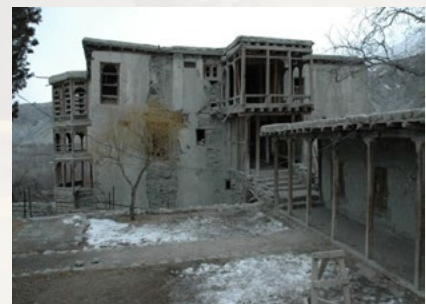
Fig 3 Khaplu Place realignment of leaned walls. Source AKCSP
