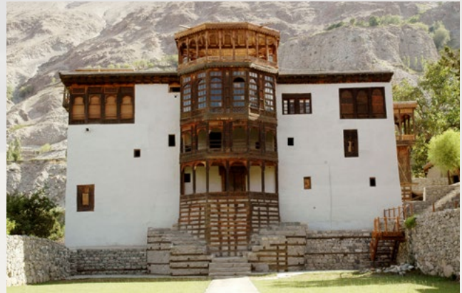
Fig 4 Post Conservation façade of Khaplu Palace
