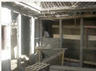
Fig 2: Decay of wooden elements
